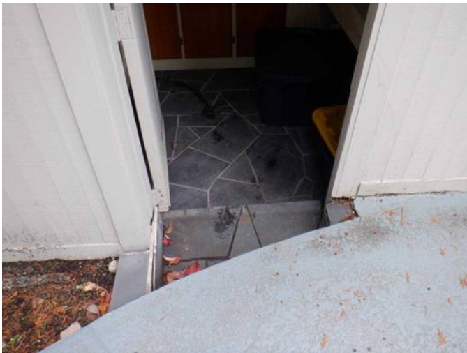
#63 Door to outbuilding bathroom opens over step down, fall hazard.
