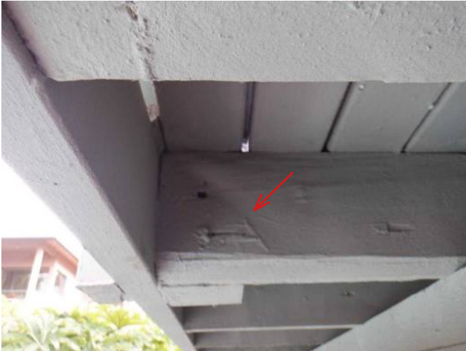
#15 Rot occurring in sections of untreated wood joists in deck system.
