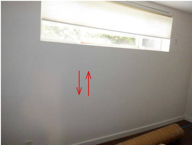
#73 Example of non egress window due to height.
