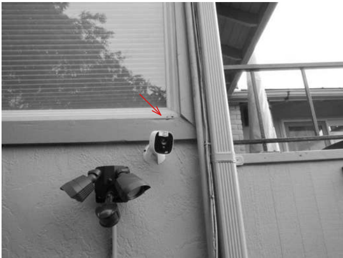
#9 Minor rot in lower SW corner of SW kitchen window trim.
