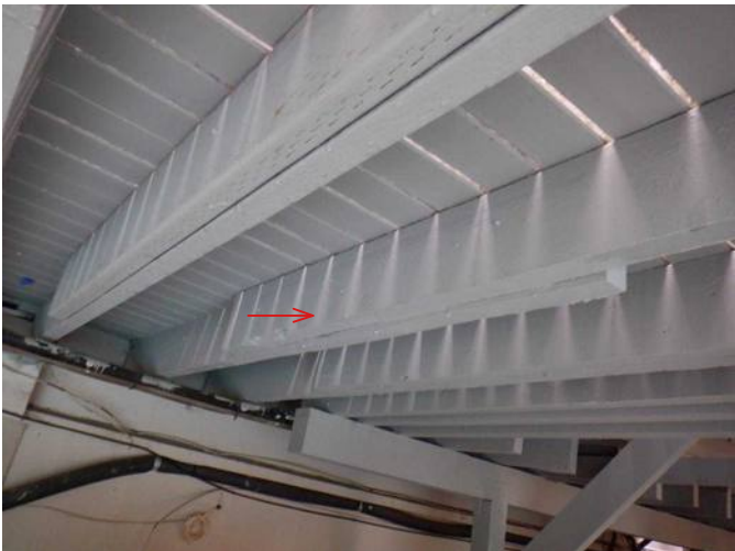
#17 A few joists are sistered mid span, need to be through bolted for stability.
