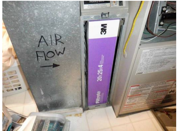
#44 Older electronic air filter for furnace has been abandoned and replaced with disposable paper filter.
