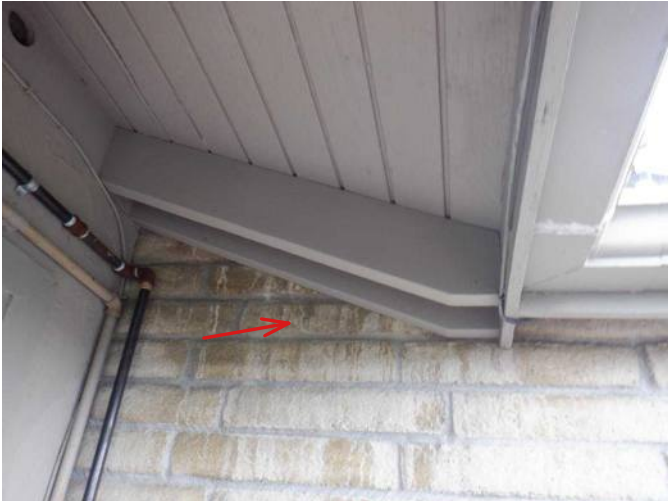
#27 Staining on chimney, at W balcony level, indicates past moisture intrusion.
