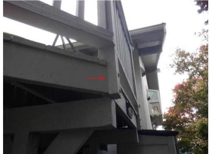
#14 Notched 4x4 railings should be replaced with full 4x4's for increased lateral strength.
