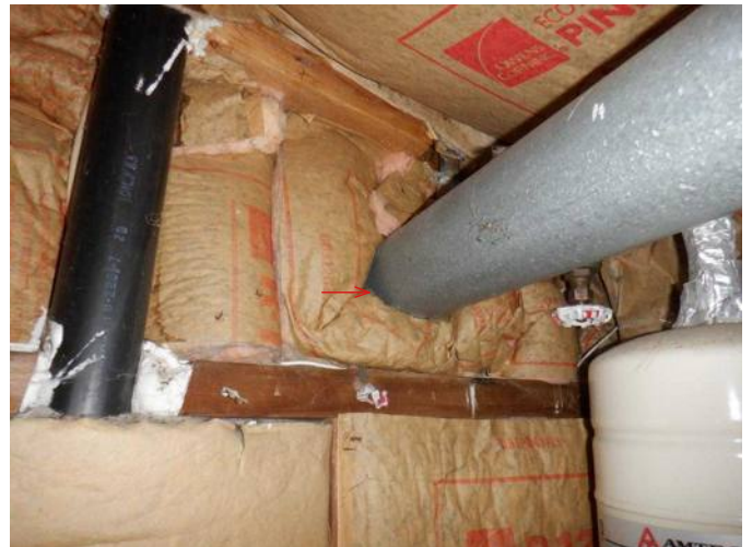
#60 Insulation in contact with outbuilding water heater flue.
