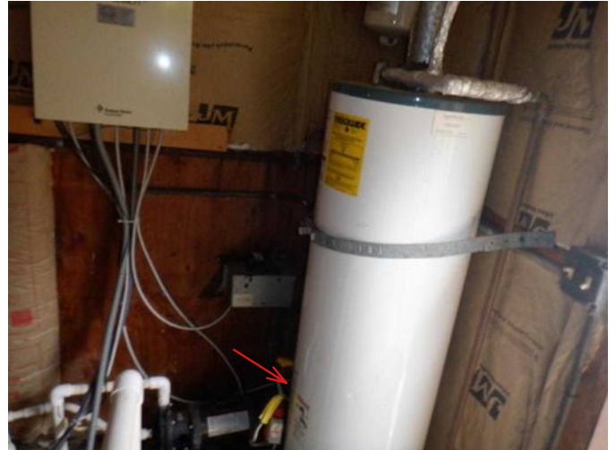
#58 No lower earthquake strap for outbuilding water heater.
