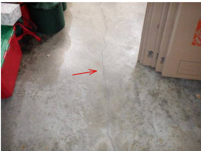
#47 Cosmetic cracks present in garage floor, normal for age of house.
