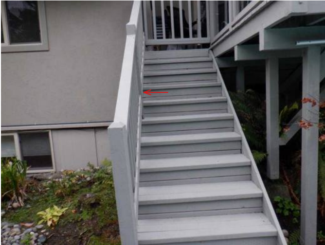
#19 Grasable handrail not installed on deck access steps.
