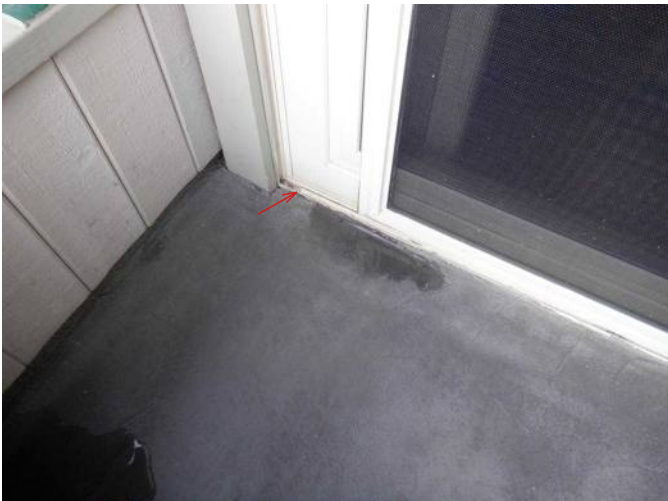
#29 Balcony surface connection to house will need to be maintained against moisture intrusion.
