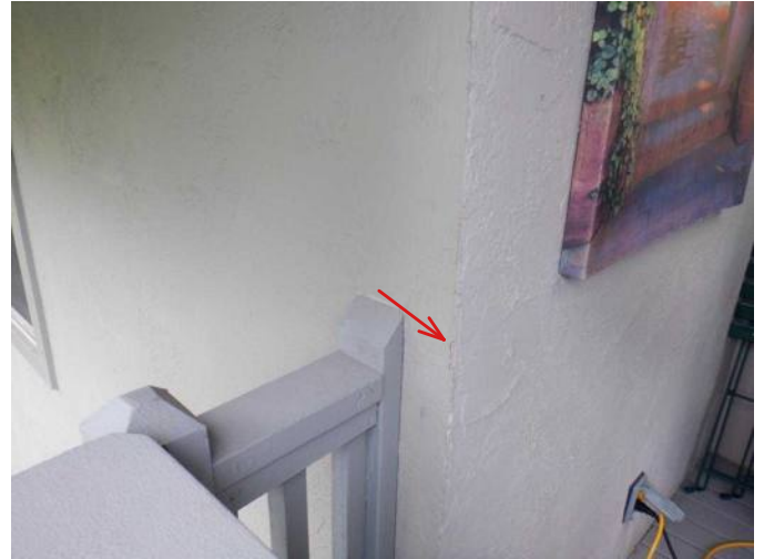
#20 Minor chipping in N stucco, visible on deck.
