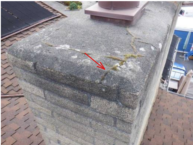
#39 Cracks in crown needs to be sealed against moisture intrusion.
