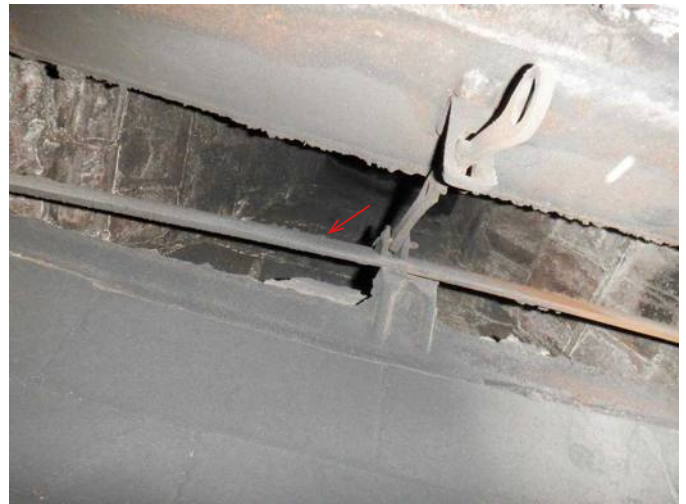
#70 Safety clamp not installed on living room fireplace damper.
