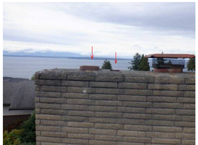
#42 Recommend rain caps be installed.
