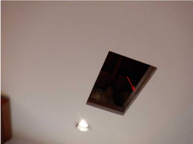
#51 No air seal present for lower attic access hatch.
