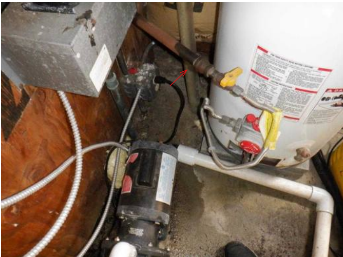
#59 No sediment leg for gas line to outbuilding water heater.
