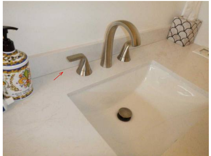
#68 Caulking needs to be redone at counter/back splash junction in first floor hall bathroom.
