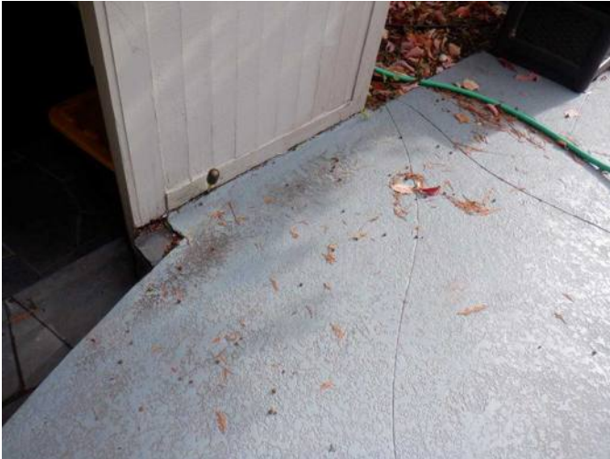
#57 Rot in lower W siding and trim of outbuilding.
