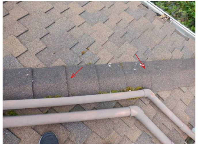
#36 Minor tears in NE hip ridge caps.
