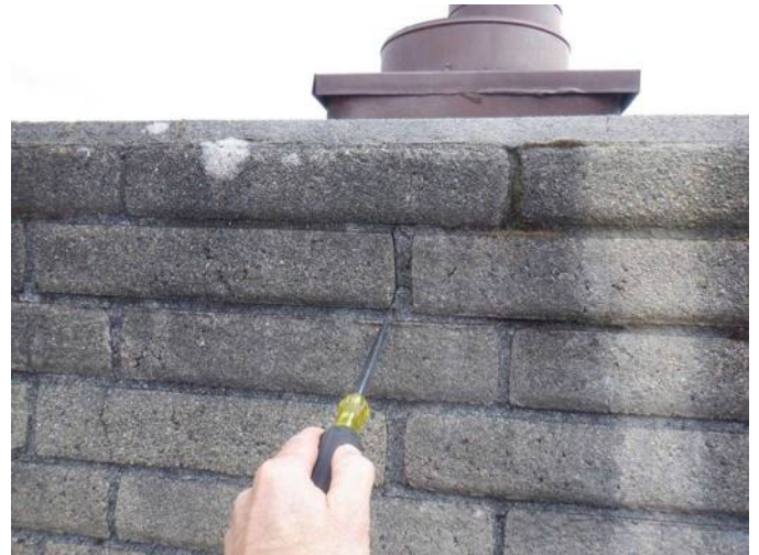
#40 Minor cracks in chimney mortar, need to be sealed.
