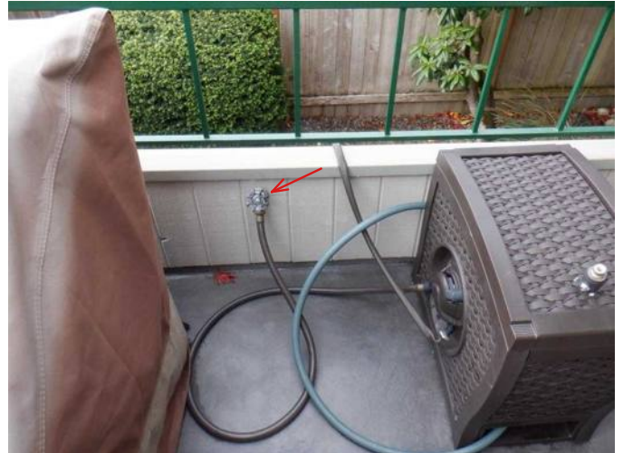
#28 Exterior W and N hose bibs do not have vacuum breakers installed.
