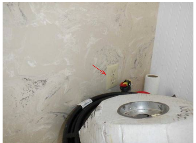
#66 Outlet in outbuilding bathroom is not GFCI protected.
