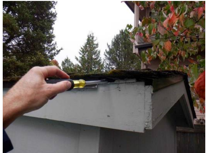
#62 Rot in SW fascia of outbuilding, drip edge flashing not installed.
