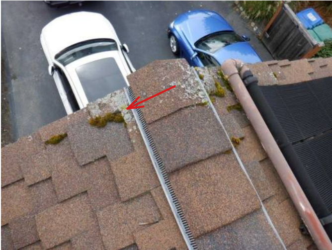
#33 Minor moss build up should be removed and moss will need to be maintained off of roof surface.
