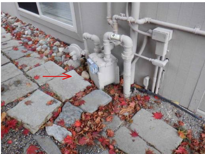
#11 6 inches of air space required under gas meter.
