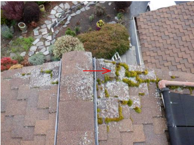
#35 Minor moss build up should be removed and moss will need to be maintained off of roof surface.
