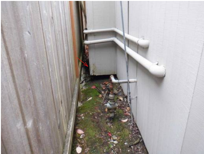
#61 Rot in lower siding of outbuilding.
