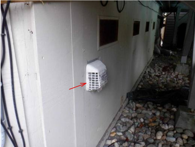
#21 Pest cage installed on exterior of dryer vent will need to be observed and cleaned when needed.
