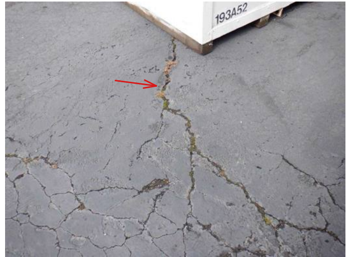
#2 Sections of driveway surface cracked.
