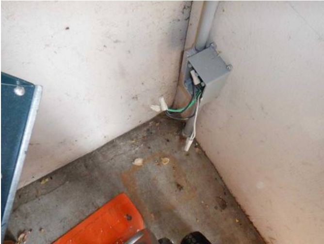
#49 Open junction box in SE corner of garage needs a cover plate.
