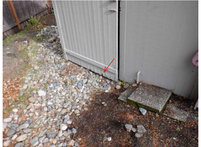
#56 Minor rot occurring along lower edge of access doors.
