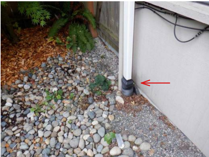
#23 Plastic corrugated pipe used as leader system has a higher potential for clogging, will need to be maintained.
