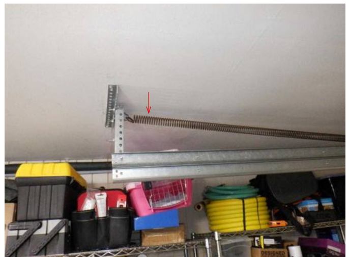
#48 Safety cables are not installed in older door springs for garage doors.
