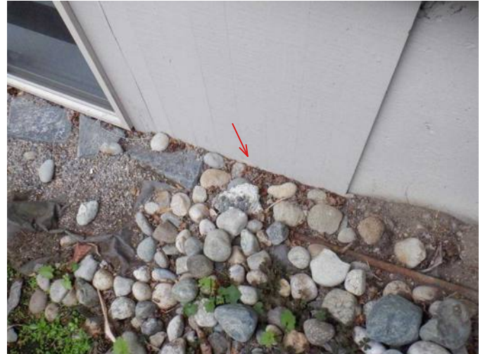
#22 Siding/soil contact along N side of house.
