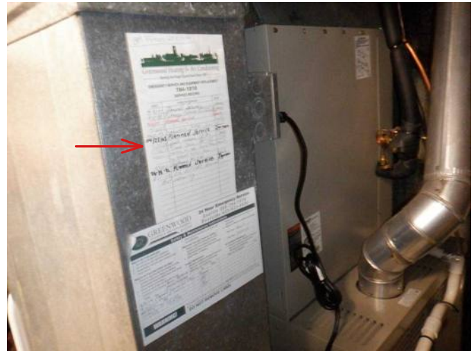
#74 Furnace is in latter third of normal life span.
