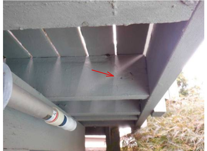
#16 Rot occurring in sections of untreated wood joists in deck system.
