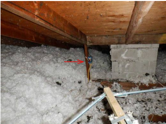
#53 Open junction boxes in lower attic need cover plates.
