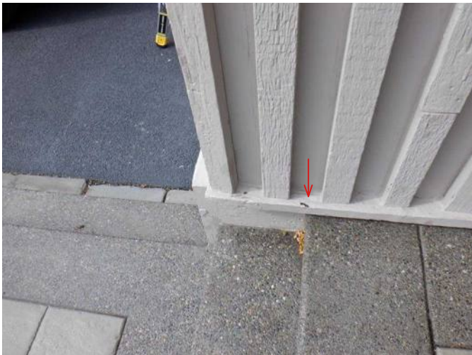
#3 Minor paint peeling in trim work.
