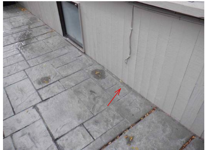
#24 Siding/concrete contact along E side of house.
