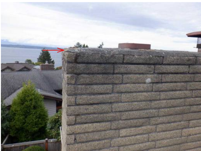
#41 Crown partially detached from chimney.
