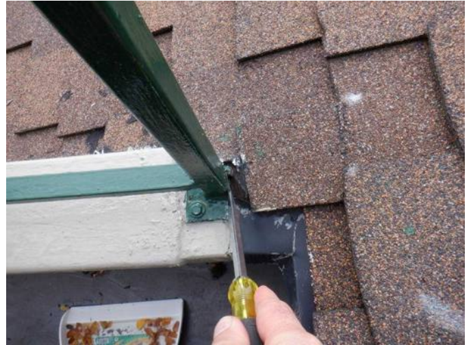
#32 Roof junction with SW corner of SE balcony relying on caulking for weather seal, will need to be maintained.
