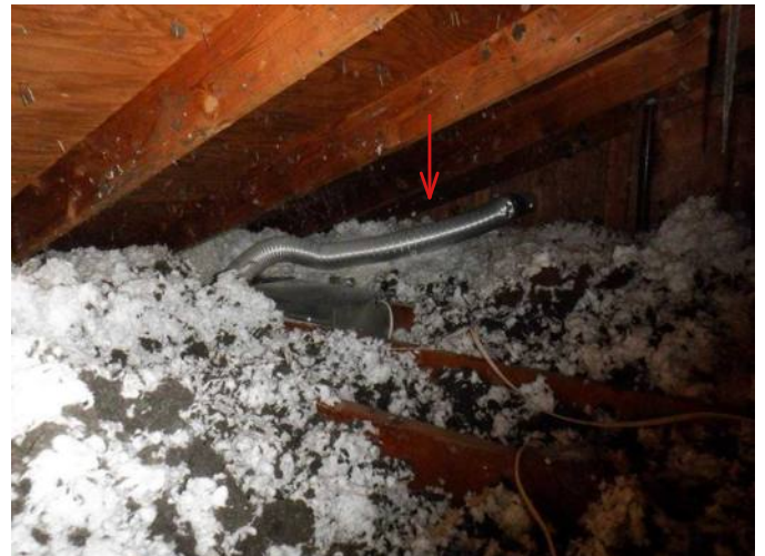
#54 Bathroom fan duct should be insulated in upper attic to reduce condensation build up in fan duct.
