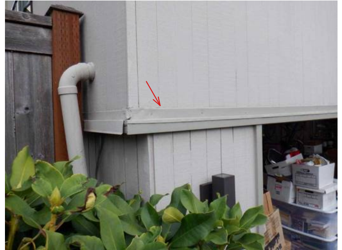
#50 High moisture reading in garage wall at this location.
