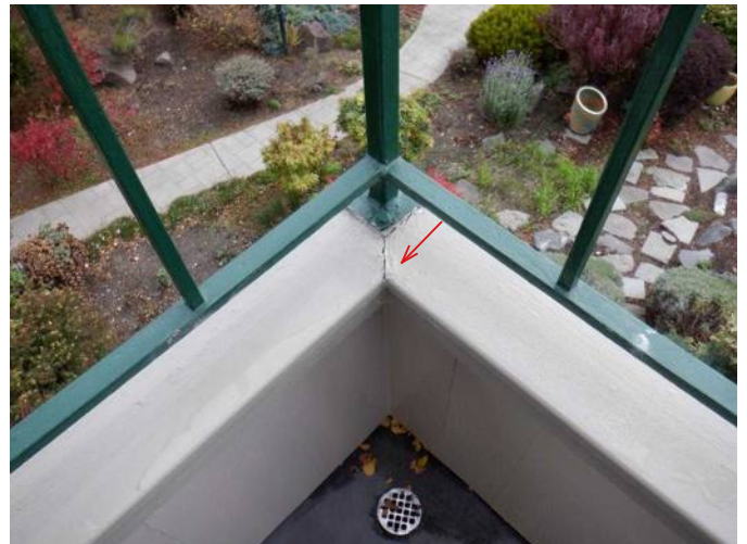
#30 Miter cut in SE balcony top rail needs to be sealed against moisture intrusion.
