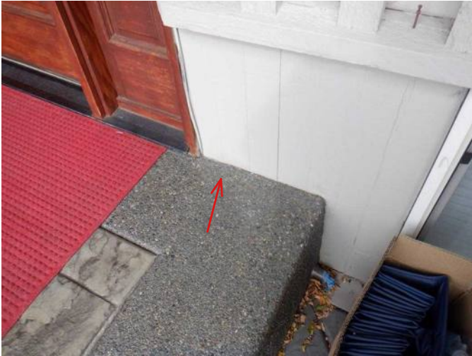
#25 Siding/concrete contact at front porch.
