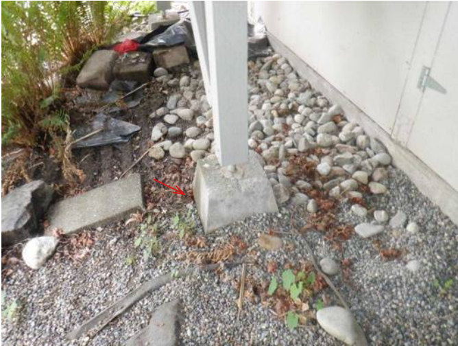
#13 Deck installed on 1X1' pier blocks, should be poured footings.
