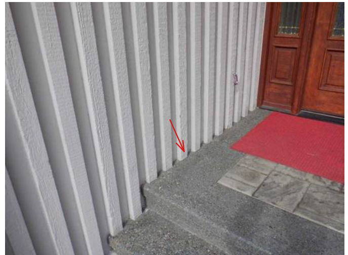
#4 Siding/trim in contact with front porch cement.
