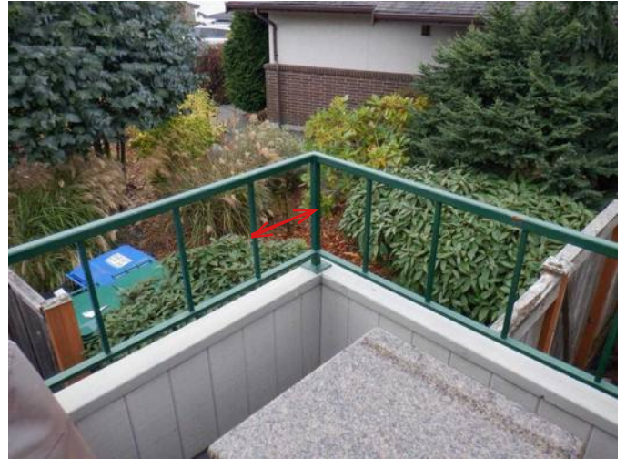
#26 Baluster spacing too wide on both balconies (safety).
