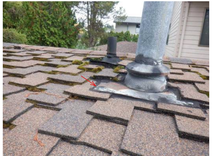
#64 Tar installed around water heater flue and plumbing vent.
