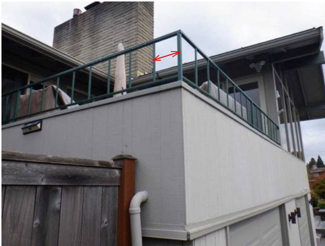
#7 Baluster spacing too wide on both balconies (safety).
