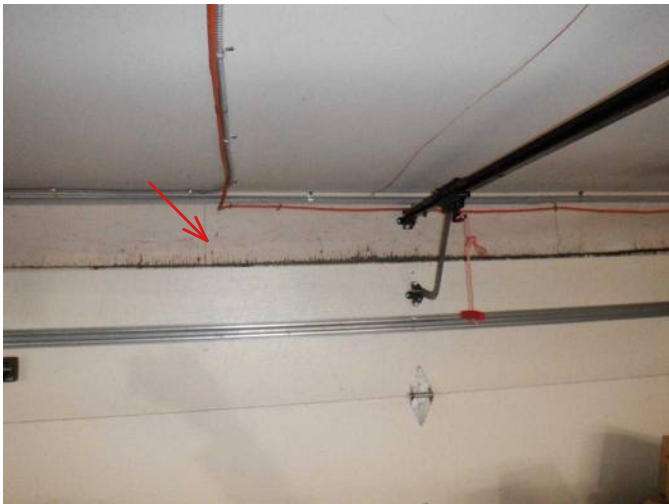
#45 Rot occurring in upper SW wall paneling over W garage door.
