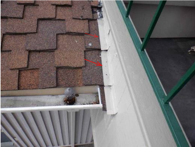
#31 Step flashing at roof/SE balcony junction, installed on top of roof material.
