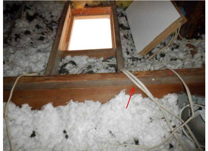
#52 Wiring installed too close to lower attic access hatch (safety).
