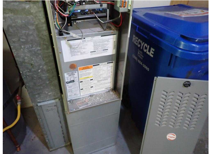
#44 No evidence of regular servicing. Furnace needs to be serviced and cleaned.
