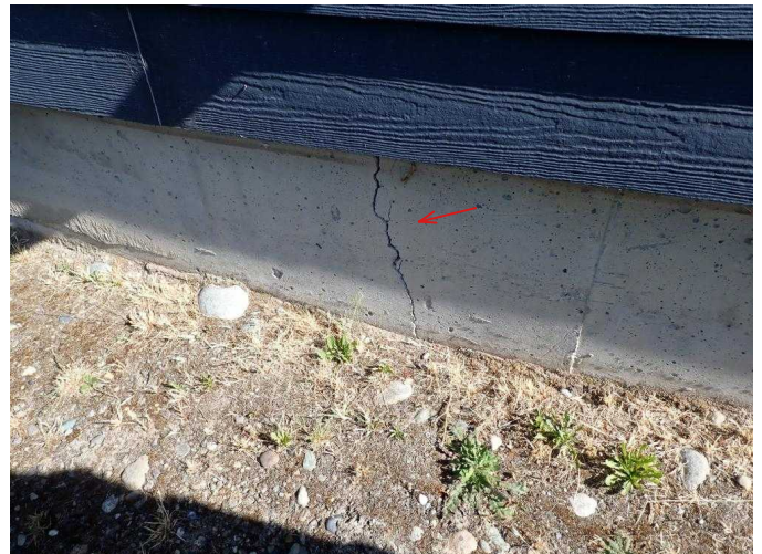
#24 Minor crack in S foundation, mid span.
