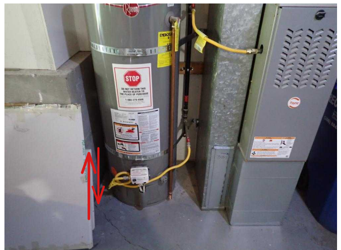
#42 Safety barrier needs to be installed in front of gas appliances to prevent potential auto impact into gas supply lines.
