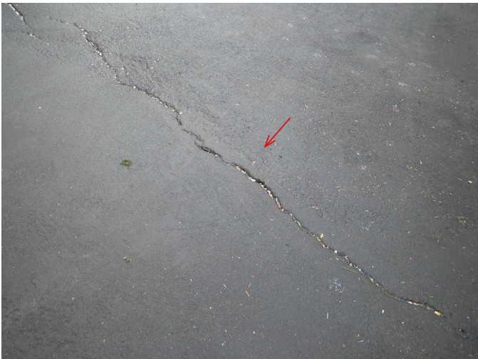
#27 Moderate cracks with moderate settling in driveway.
