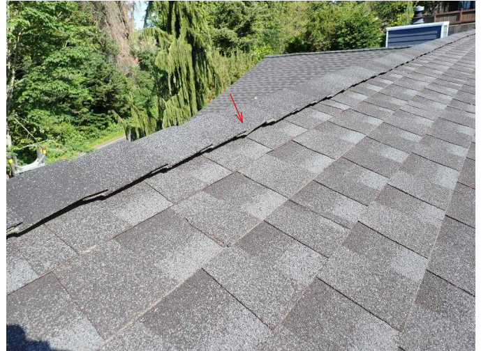
#32 Type of ridge vent installed, internally baffled, has been shown in testing to have a reduced air flow potential.
