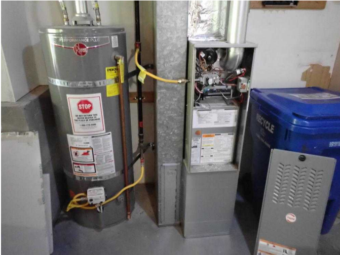
#43 Water heater and furnace in garage.
