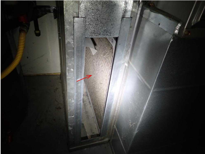
#45 Furnace filter is dirty, needs to be changed.
