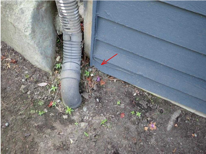
#7 Minor rot in lower NW siding where in contact with soil, soil needs to be removed.
