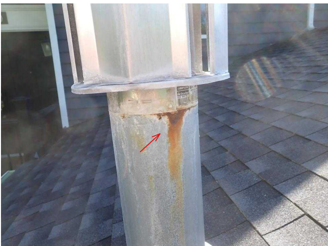
#29 Exterior section of furnace flue starting to rust and will need to be replaced in next 5 years.
