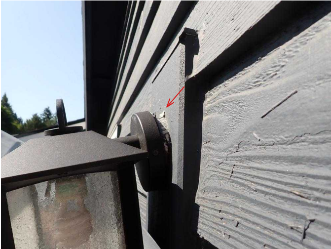
#13 Deck light fixture partially detached from base.
