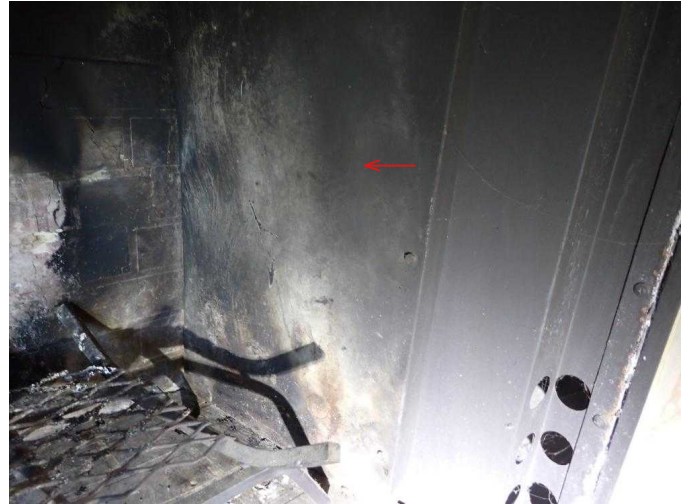
#50 Minor warping in side panels due to overheating.
