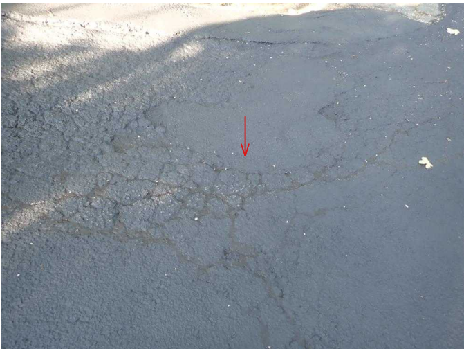
#3 Moderate cracks with moderate settling in driveway.
