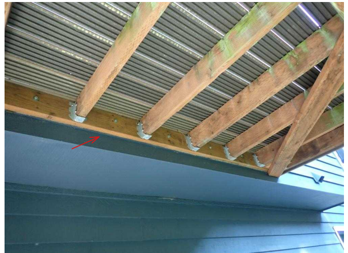
#18 Balcony installed to cantilever of house, vertical load of balcony needs to be supported.
