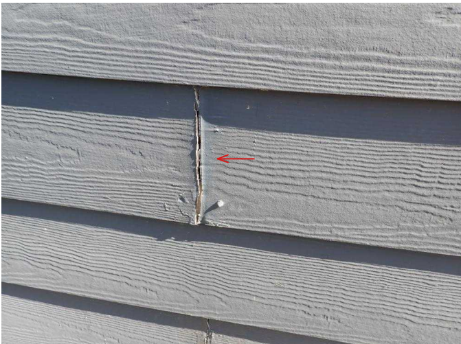
#23 Caulking cracked at some butt joints, needs to be resealed.
