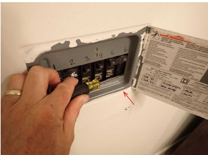
#59 Secondary electric panel is not installed flush with sheet rock causing a gap between the breakers and the panel cover.
