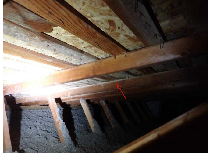
#64 Appearance of possible light vegetative haze on sections of original skip sheathing material.
