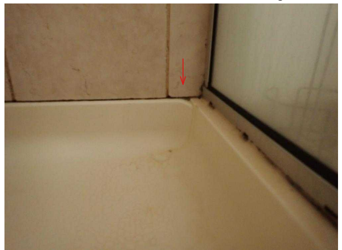
#54 Weep holes at base of primary shower surround at junction with shower pan next to door have been sealed.
