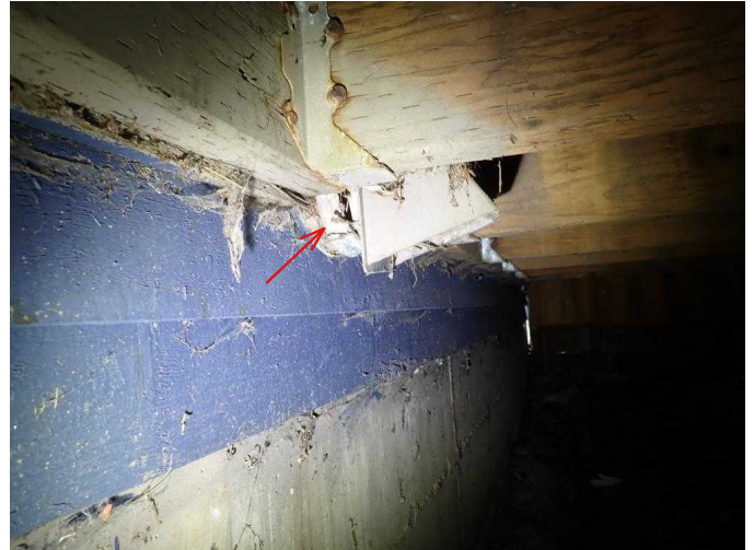
#16 Abandoned exhaust vent under deck should be sealed.
