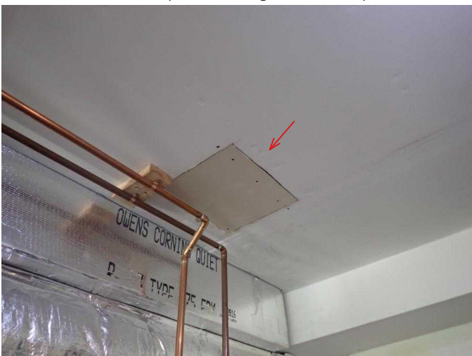
#41 All open gaps and holes in garage ceiling need to be sealed against fire intrusion.
