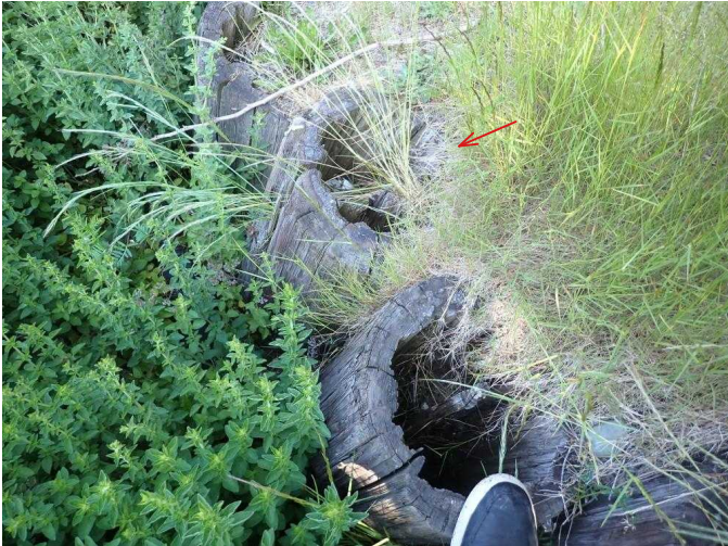
#21 Rot occurring in lower S wood retaining wall.
