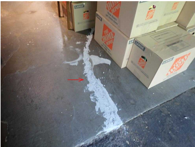
#39 Heavy crack with minor settling in SW section of floor. Crack indicates past settling, has been patched.
