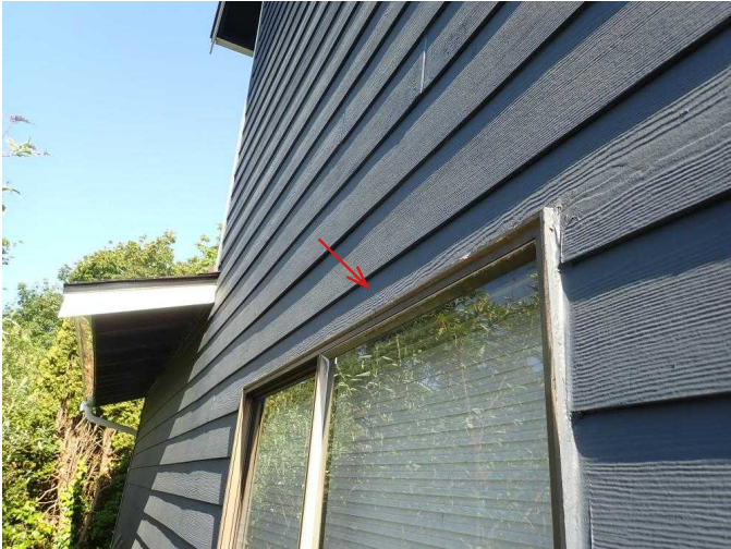
#25 No head flashing over S window.
