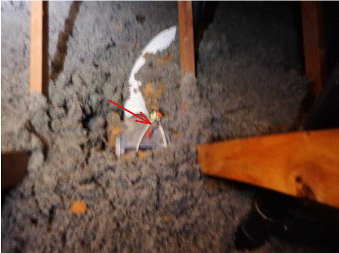
#63 Exposed wire splices at bathroom fans need to be in junction boxes.
