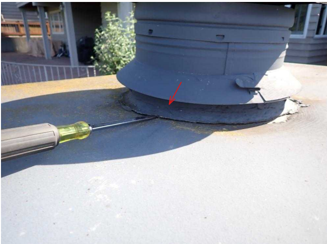
#35 Weather seal cracked around flue cap, potential water intrusion spot.
