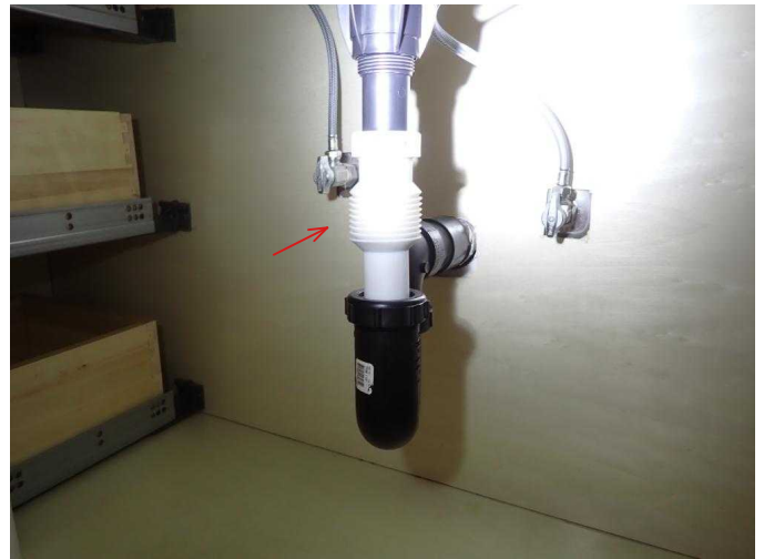
#52 Flex type drain line should be replaced with solid type drain line to reduce risk for failure/leakage.
