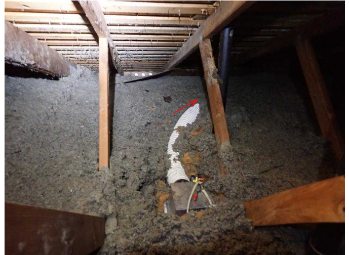
#62 Bathroom fan vents exhaust near soffit vents, need to be sealed to exterior.
