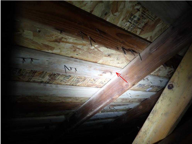
#61 Appearance of possible light vegetative haze on sections of original skip sheathing material.
