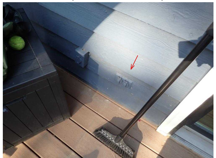
#12 Deck outlet is not GFCI protected, all exterior outlets should be GFCI protected.
