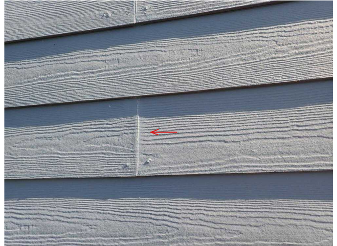
#22 No flashing at concrete lap siding butt joints, caulking will need to be maintained.
