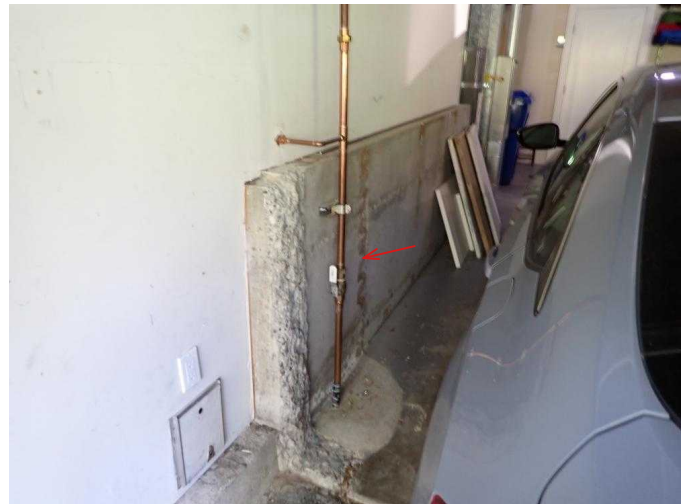
#40 Main water shutoff located on N wall in garage.
