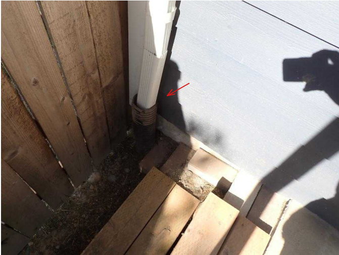
#19 Corrugated leader pipes will have a higher potential for clogging and will need to be maintained.
