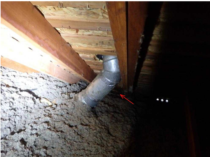
#65 Kitchen fan vent should be insulated to reduce condensation.
