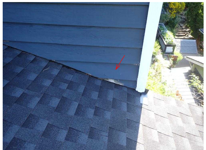
#30 Minor paint peeling on upper W siding at connection to garage.
