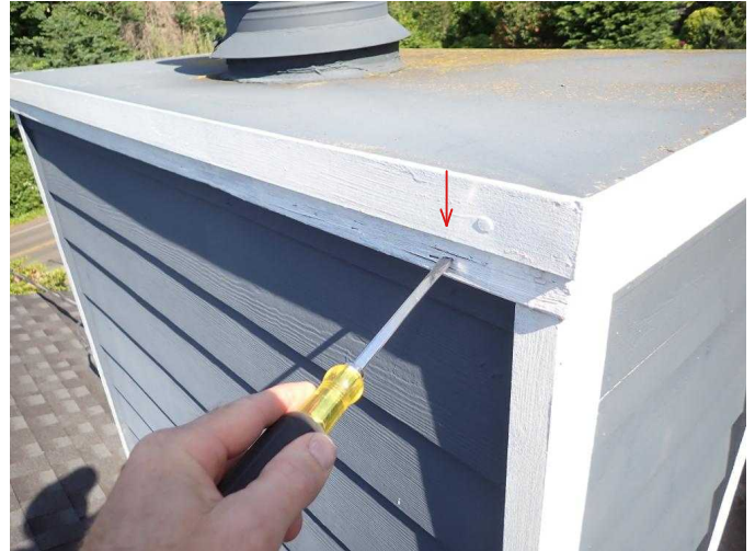
#34 Minor rot in upper trim of chimney.
