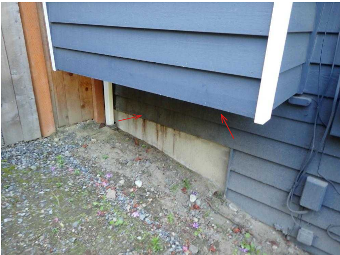
#9 High moisture reading in house siding underneath chimney and in soffit of chimney.
