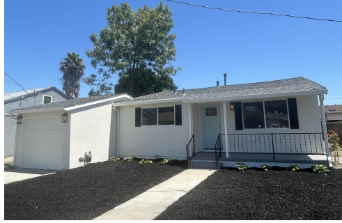
Front Of Structure
